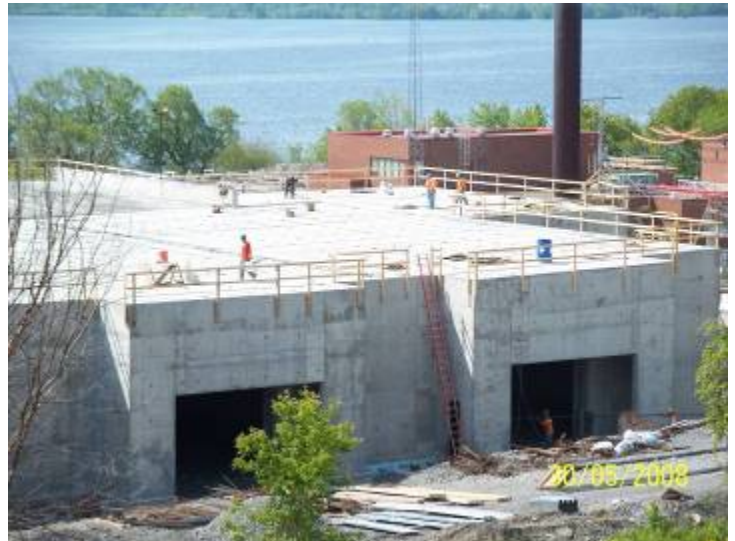
Biosolids Storage Facility: The pre-cast Concrete roof has been installed on this building. The biosolids will be stored in this facility until it can be applied to farm fields. The building will be fully enclosed with an odour control system to minimize odours, one previous concern of everyone.
