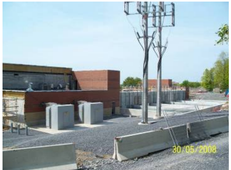
Biosolids Storage Facility: The pre-cast Concrete roof has been installed on this building. The biosolids will be stored in this facility until it can be applied to farm fields. The building will be fully enclosed with an odour control system to minimize odours, one previous concern of everyone.
